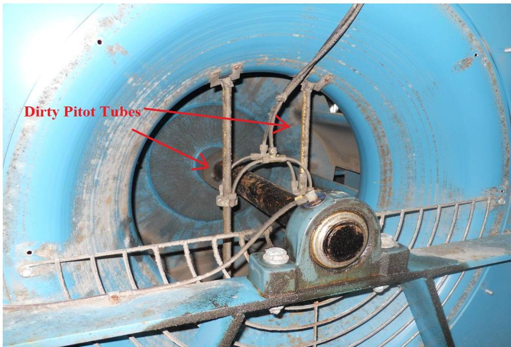
With the dirty pitot tubes reading a higher airflow on the supply side the return fan in turn ran at a higher speed to try and maintain the same return airflow. This resulted in excess fan energy and an unbalanced space with airflow and pressure. Simply cleaning the tubes allowed the airflow station to read a lower accurate airflow and the fan VFDs were able to ramp down which saved energy and produce a better-balanced space.
